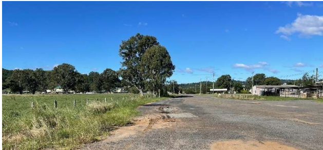
Figure 1.16: View looking east along Alexandra Parade toward the Showground (Source: EJE Architecture)
