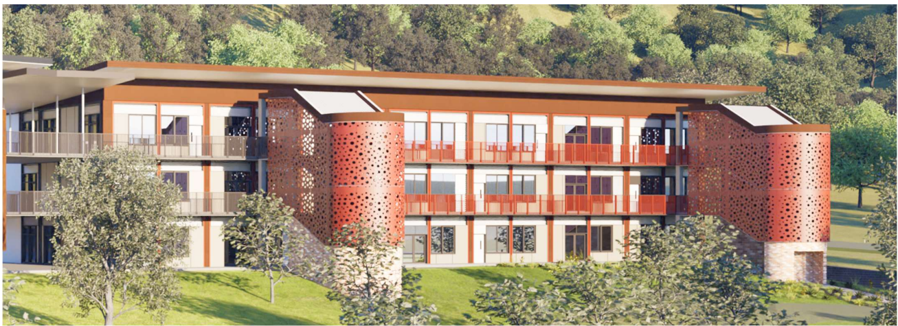
Figure 7.05: Render of Building D showing connection to Building C (Source: EJE Architecture)
