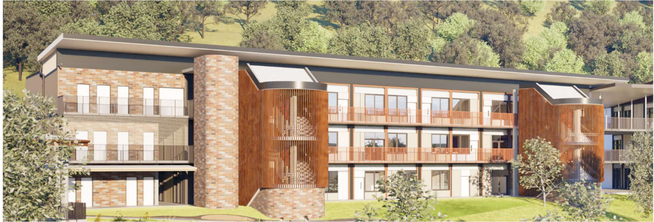
Figure 7.04: Render of Building C showing vertical circulation cores and connection to Building D (Source: EJE Architecture)
